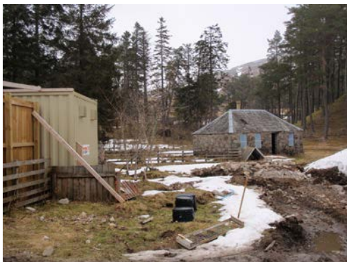
Fig. 9 : Existing cottage to be demolished
